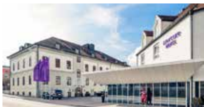
Mercure Hotel München Airport Freising (I)
